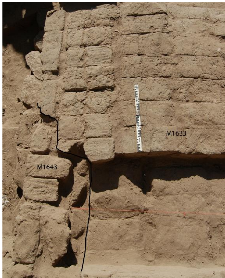
Fig. 15: Cracks in the brickwork of later town wall M1633 and repairing M1643.
