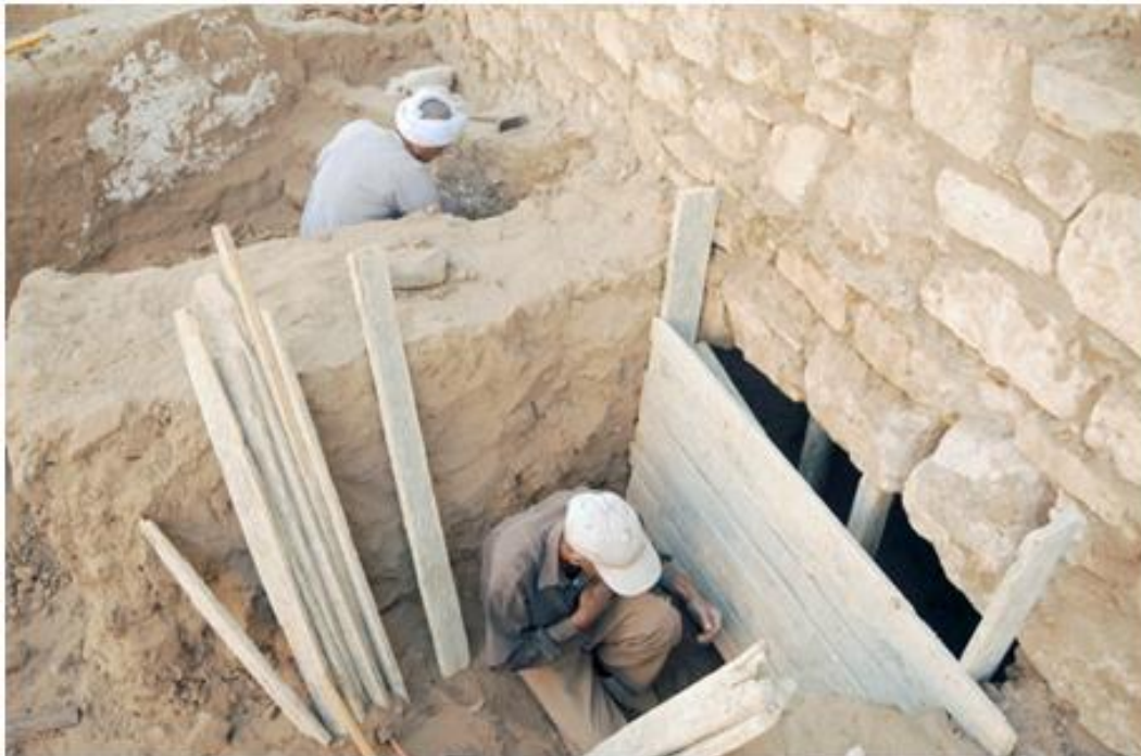
Fig. 2: Excavation and underpinning of the foundation of the old museum
